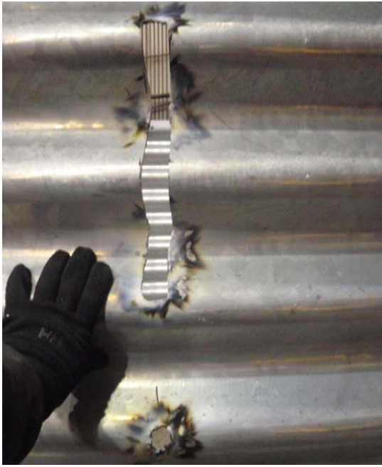
Photo 9: Close up view of slots being cut in the DN Camp Sumps.
